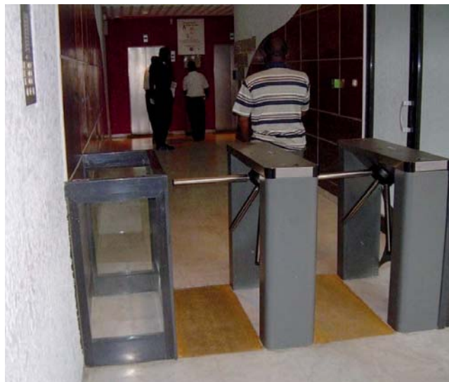
View of an access control turnstile
