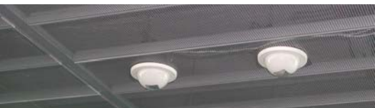
Over 100 cameras are connected to the access control system.
